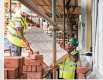
The insulation boards can be readily cut using a sharp knife or fine toothed saw. Ensure tight fitting of the insulation boards to achieve continuity of insulation as asked for within the ACDs. Appropriate PPE should be worn when handling insulation. Please refer to Health & Safety data sheets on our website.
